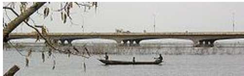
Third Mainland Bridge
