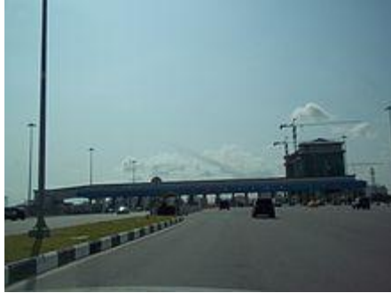
Toll gates and roads in Lagos Lekki-Epe Expressway
